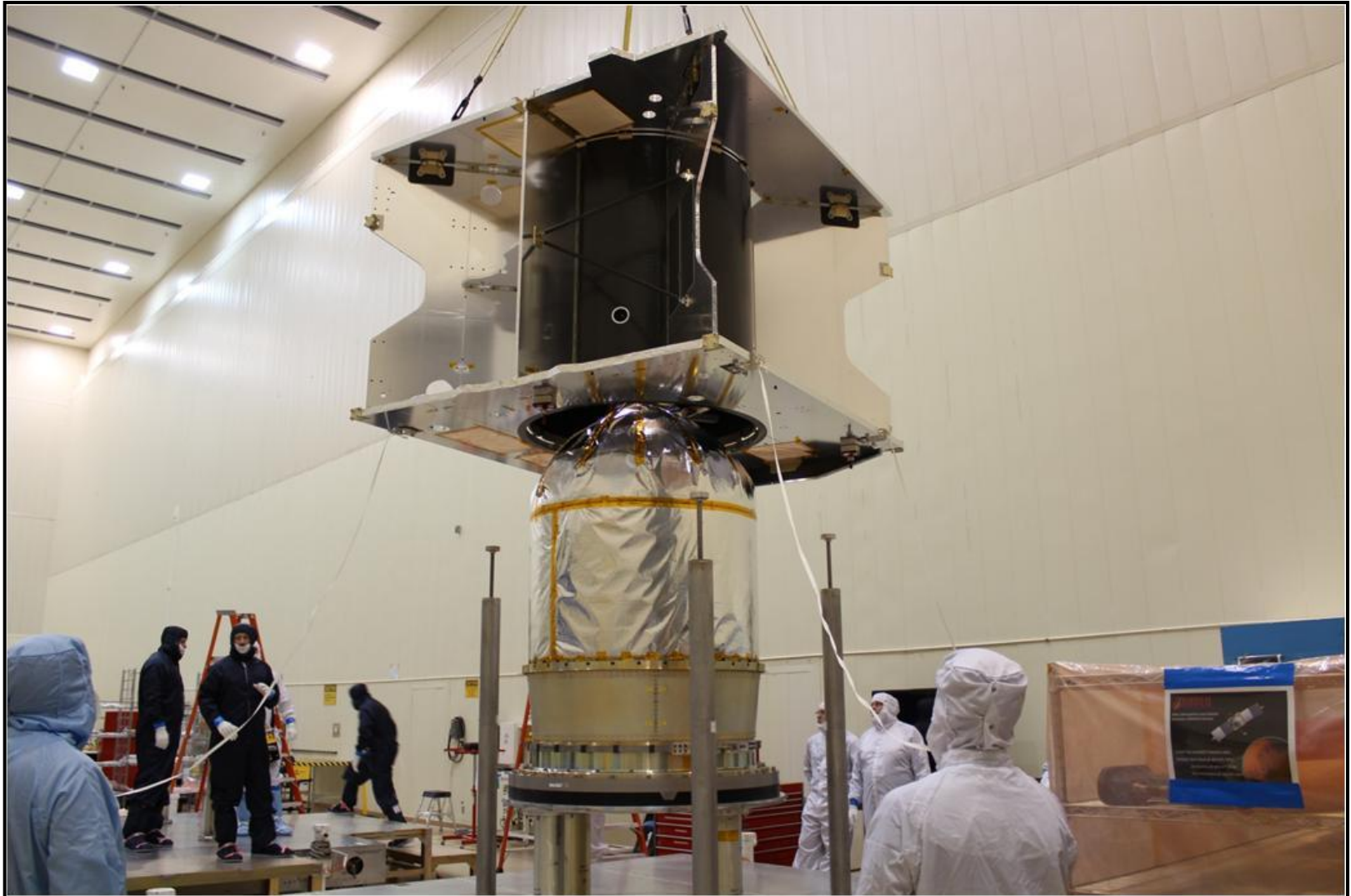
Integration of core structure with fuel tank
